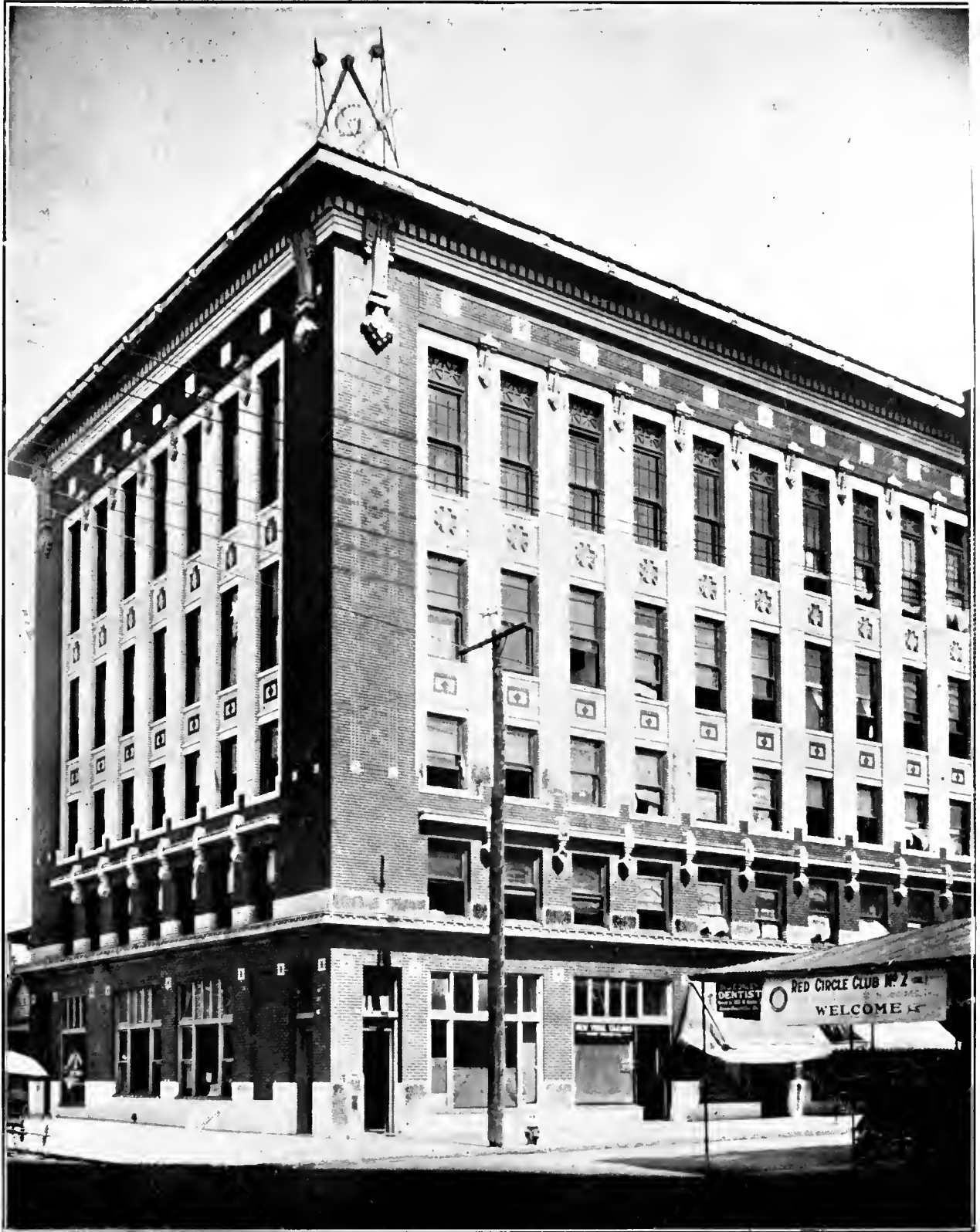
MASONIC TEMPLE BUILDING—JACKSONVILLE, FLA.
